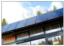
Photovoltaic panels on the roof which generate free electricity without depleting fossil fuels or giving rise to harmful greenhouse gases. There is an electronic performance display in the reception foyer
