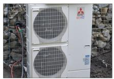
The air source heat pump which heats the building in a very efficient way. Every unit of electricity it uses is converted into four units of heat. Sophisticated controls get the heat to where it is needed most
